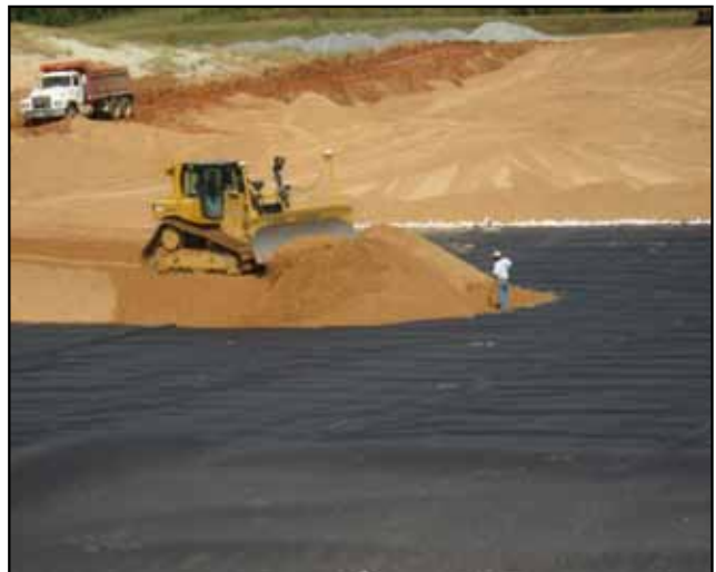
Placing Protective Cover
