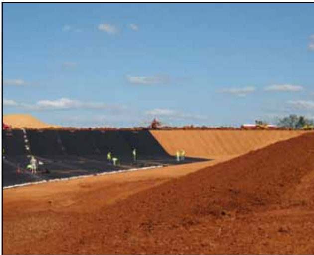
Liner Being Installed
