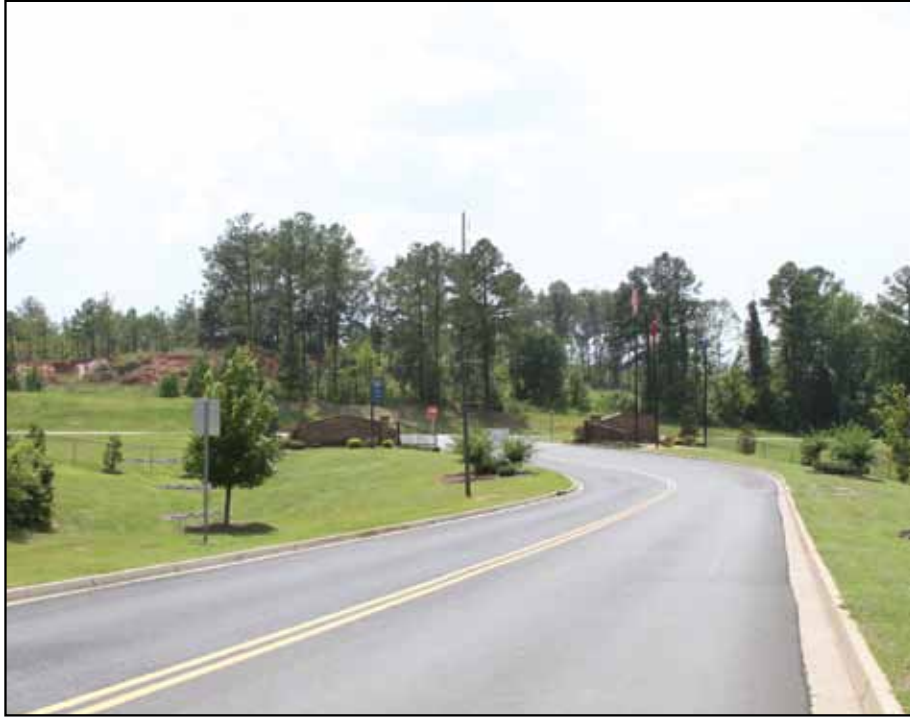
Exiting the Landfill
