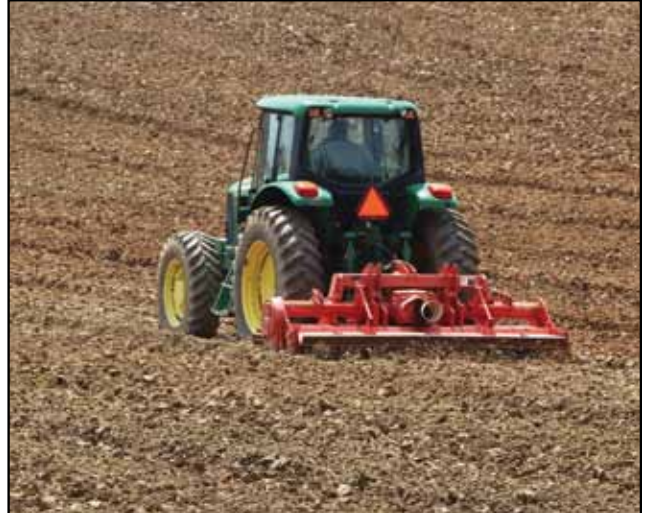
Processing Soil For Clay Liner
