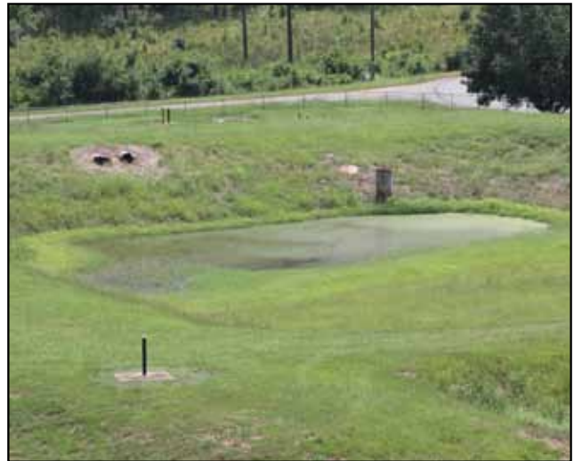
Detention Pond Phase I
