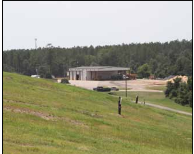
Well Field Phase II
