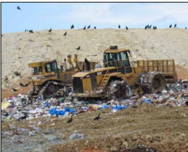
Compactor - Compacting Waste
