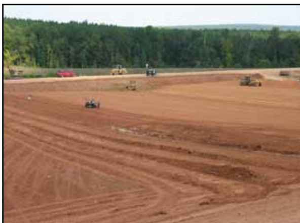
Phase IV Cells 3, 4 & 5 Construction
