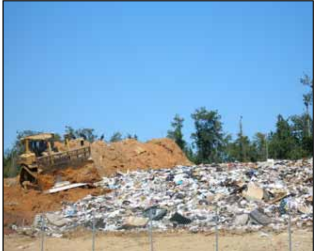
Waste Being Covered Daily
