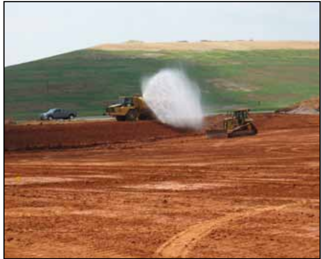
Applying Water To Clay Liner
